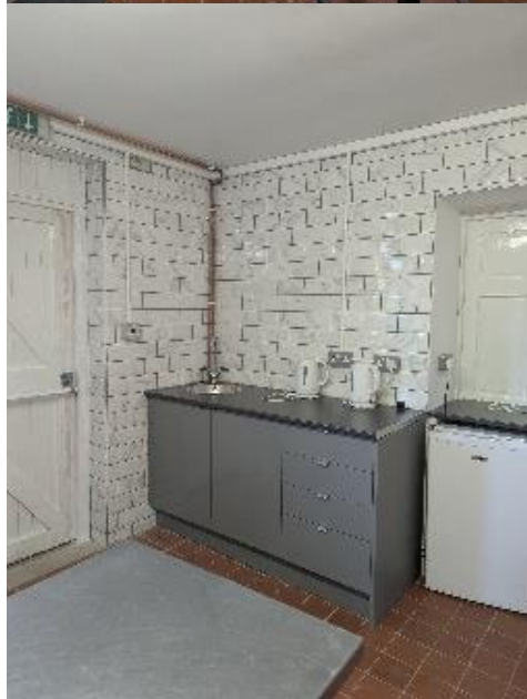
The newly refurbished village hall kitchen – see page 9
